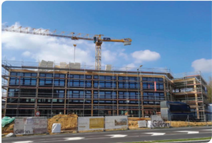
The Mundo Lab center in Louvain-la-Neuve under construction
