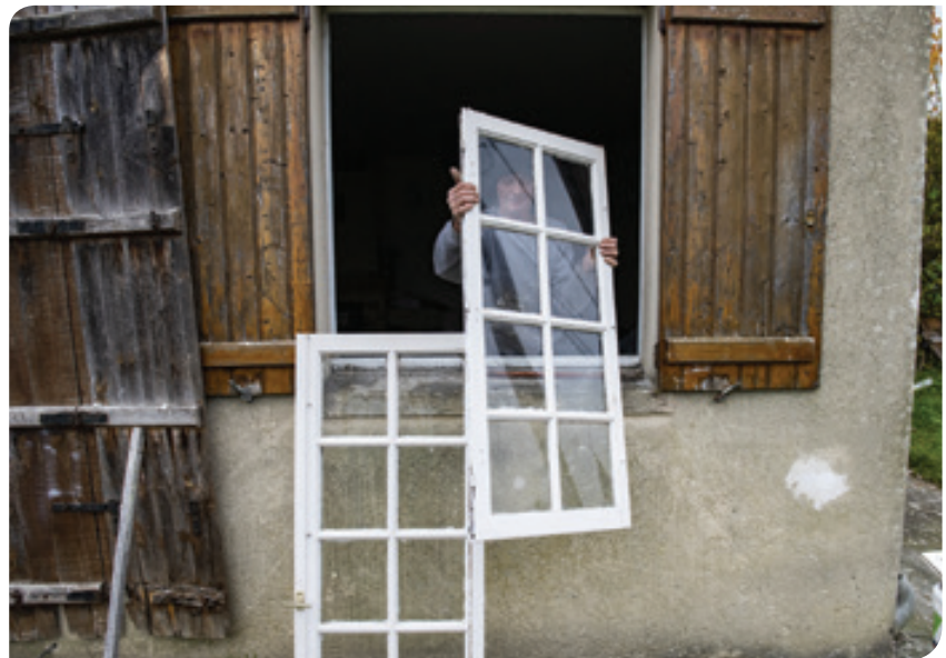
Energy renovation work coordinated by REH
